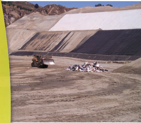
Phase 1: Landfill preparation
