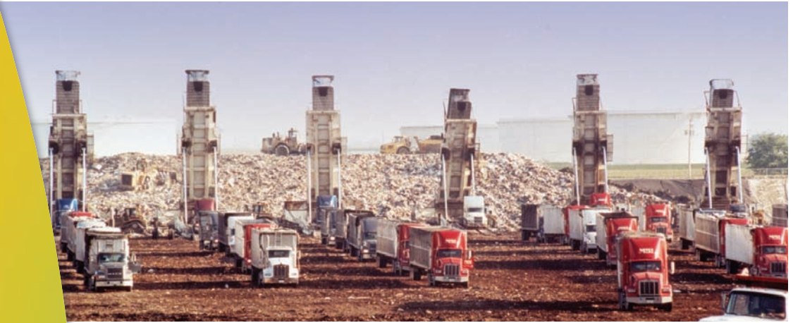
Phase 2: Working face of live landfill, Pontiac
