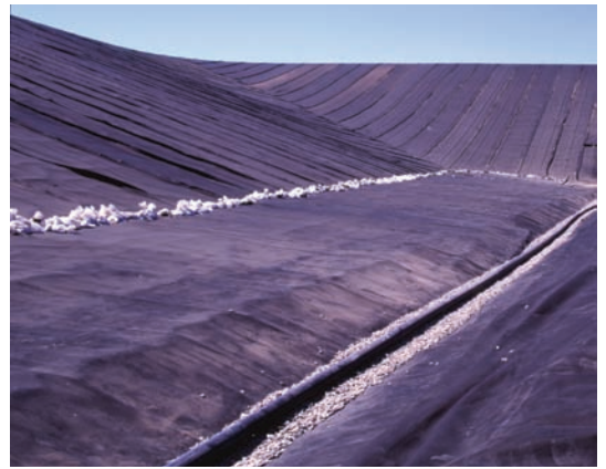
Phase 3: Capping of landfill
